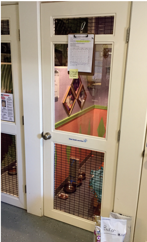
Figure 8 Individual room doors that allow viewing through a glass panel (centre of door) and interaction and ventilation through plastic-coated grates (top and bottom of door)
